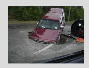
Liquefaction began to appear almost instantly after the initial earthquake. Aftershocks turned water-saturated layers of sand and silt beneath the surface into sludge that squirted up through the cracks caused by the earthquake. Streets were drowned in liquefaction damage and sewage from broken pipes.
